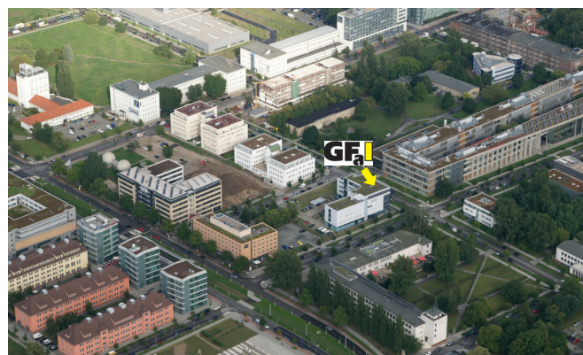
The building of the GFal in the science and technology park Berlin-Adlershof
