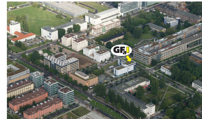
The building of the GFaI in the science and technology park Berlin-Adlershof
